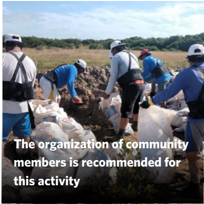
Filling and transfer of sediment and organic material to areas with a low topographic level
